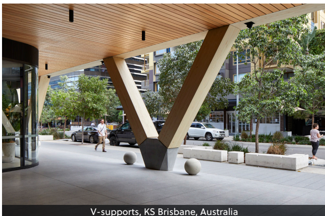
V-supports, KS Brisbane, Australia
