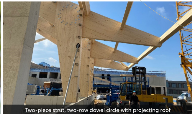
Two-piece strut, two-row dowel circle with projecting roof
