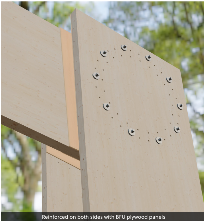
Bend-resistant frame corner with rectangular clearance profile
