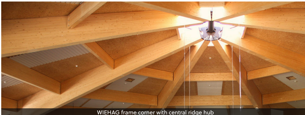
WIEHAG frame corner with central ridge hub
