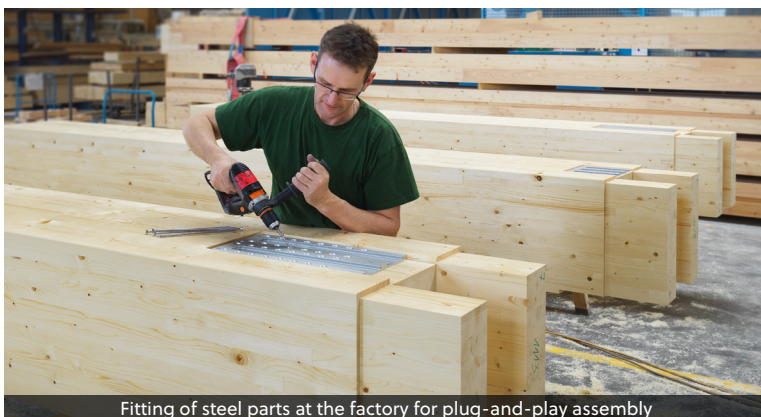
Fitting of steel parts at the factory for plug-and-play assembly
